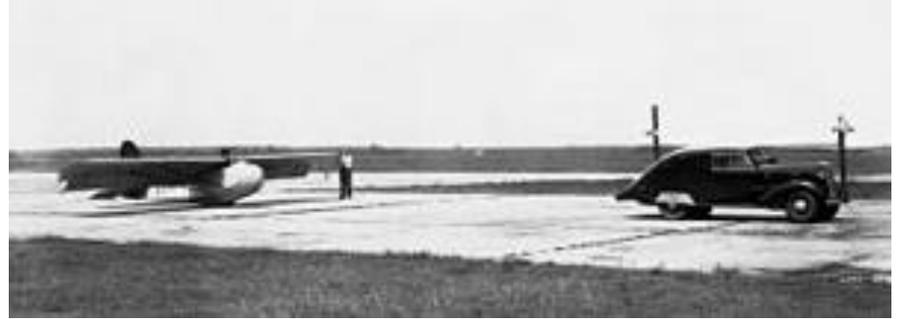
Franklin PS-2 training glider is about to be towed aloft by the specially modified car in front.
